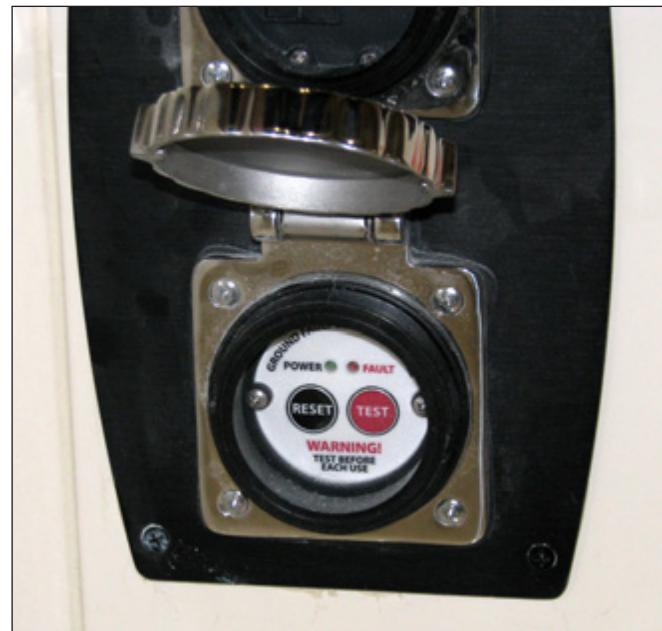
ELCI Inlet Panel & TEST/RESET Buttons
