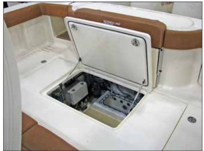
Aft Systems Room Hatch
