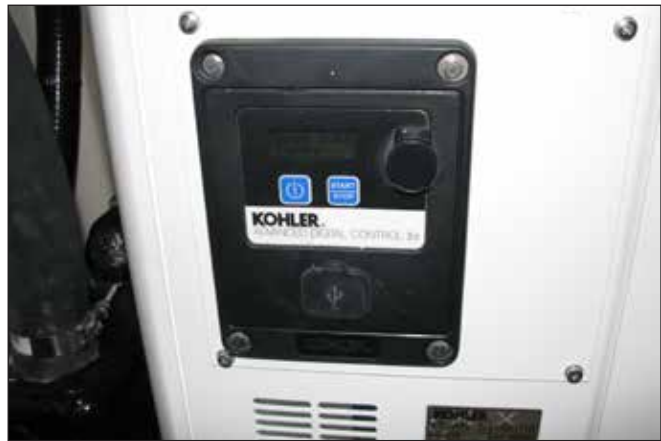
Generator Onboard Control Panel
