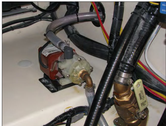
Air Conditioner Seawater Cooling Pump
