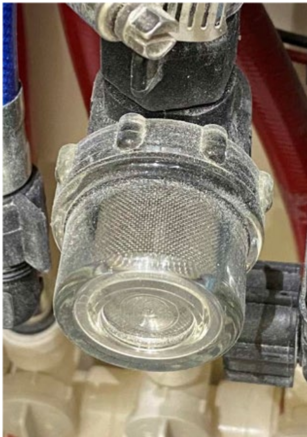
Fresh Water Pump Strainer
