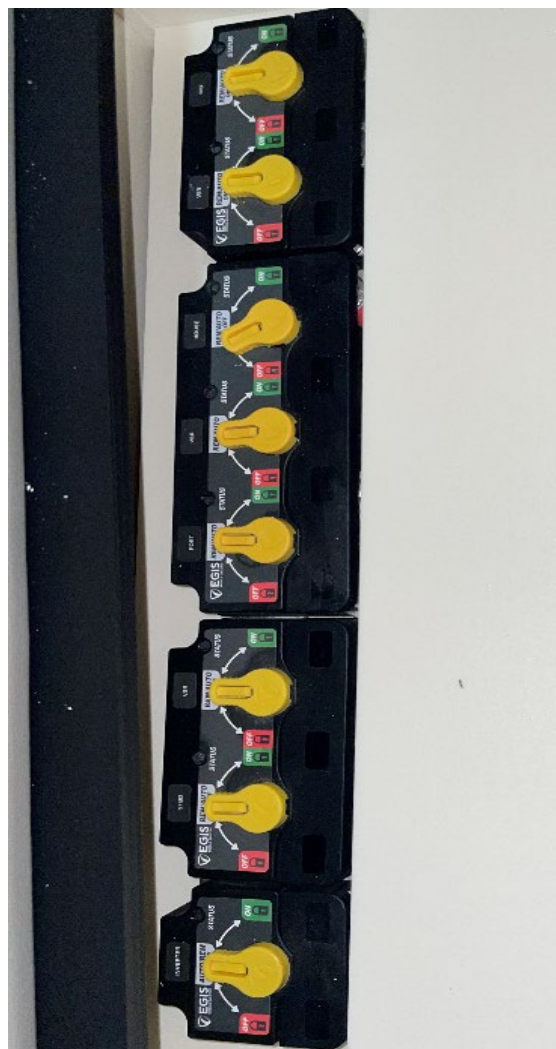
Battery Select Switches
