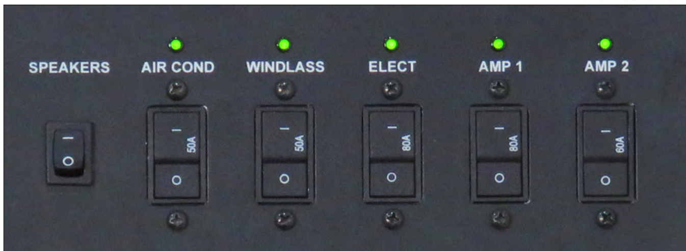
Typical DC Panel Heavy Duty, Slot Reset, Circuit Breakers
