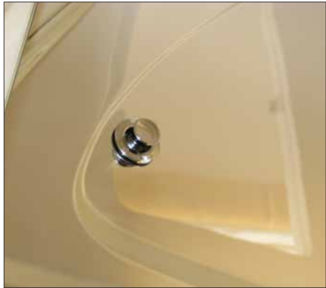
Cabinet Door Latch With Locking Mechanism Released
