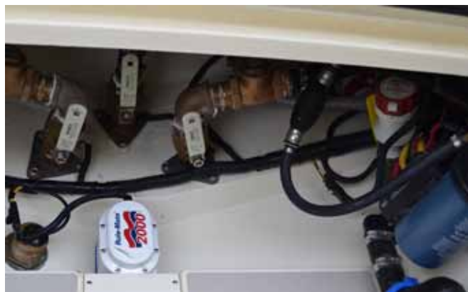
Bilge Pump and Baitwell Pumps
