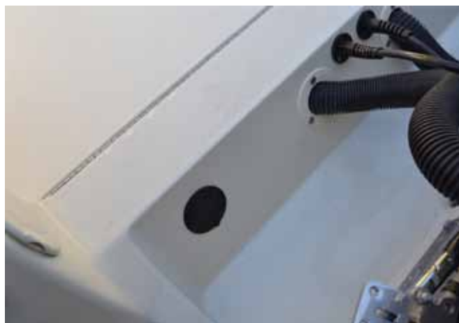
Raw Water Quick Disconnect in Splashwell
