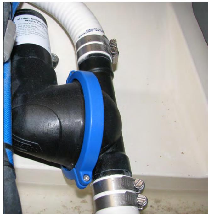
Typical Waste Discharge Diaphragm Pump
