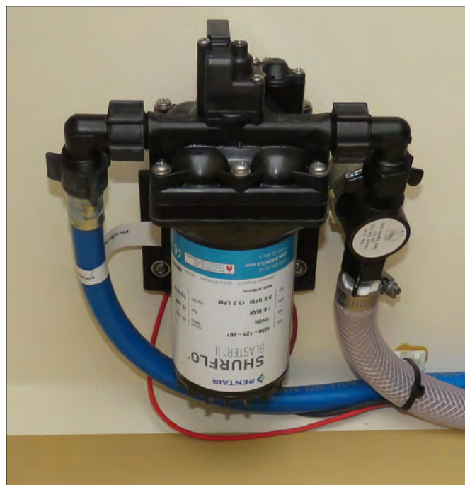
Typical Fresh Water Pump & Strainer
