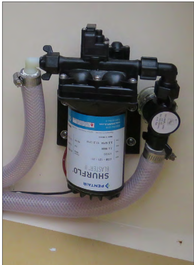
Raw Water Washdown Pump & Strainer
