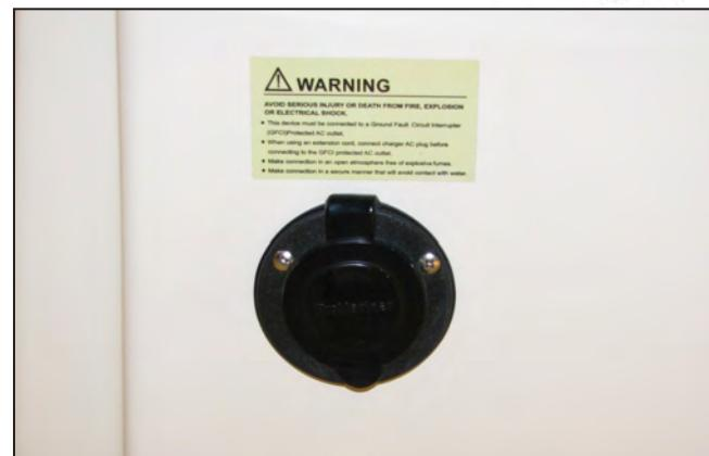
Typical Battery Charger Inlet Connection
