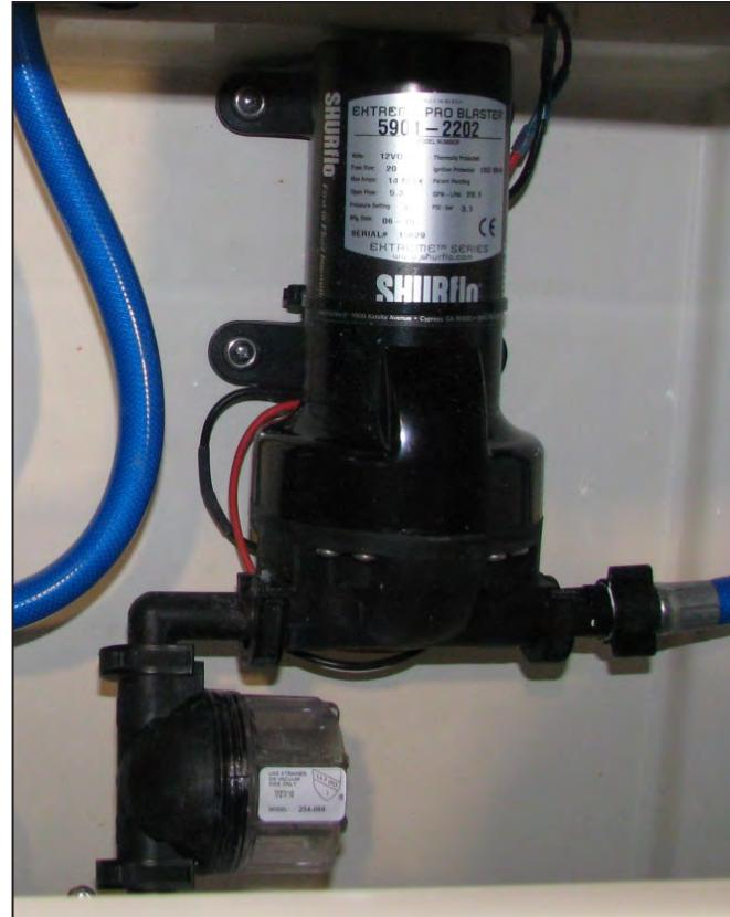
Typical Raw Water Supply Pump & Strainer
