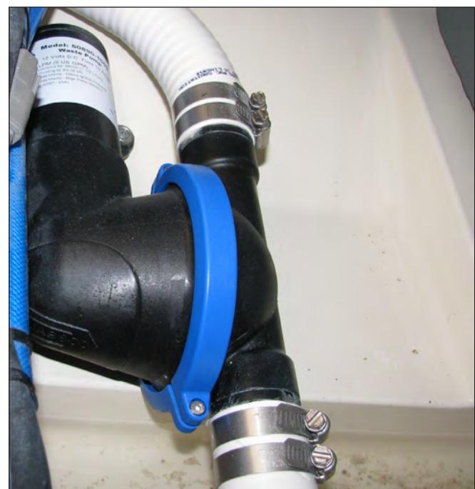
Typical Waste Discharge Diaphragm Pump
